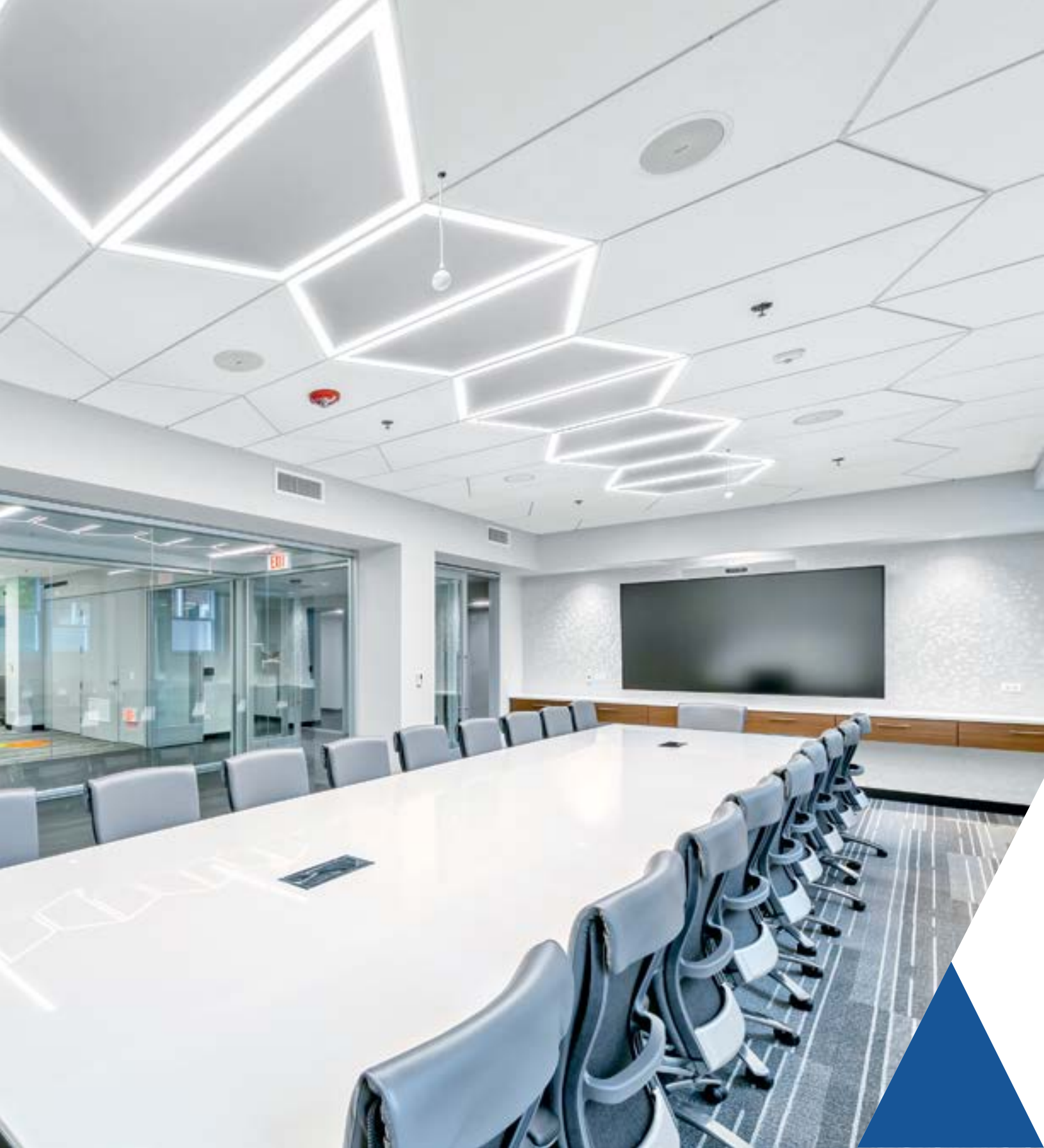
▲ Ultima® Shapes para DesignFlex®/MetalWorks™ Shapes para DesignFlex/Sistema de suspensión Suprafine® XM con Axis Sculpt Geometric Light Fixtures; Insurance Company Centro de Capacitaciones, Chicago, IL, The Interior Design Group, LTD
